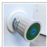
Water Supply Flow Control Valve
